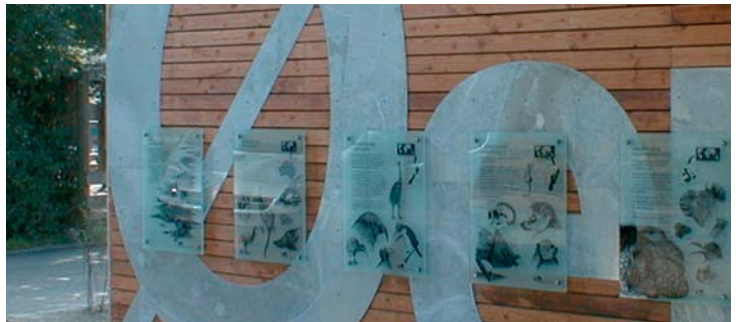
Copenhagen Zoo. Hardened, laminated glass mounted onto wood using stainless steel fittings. Reversed graphics printed on the back. Milled lettering in heat-galvanised steel.
